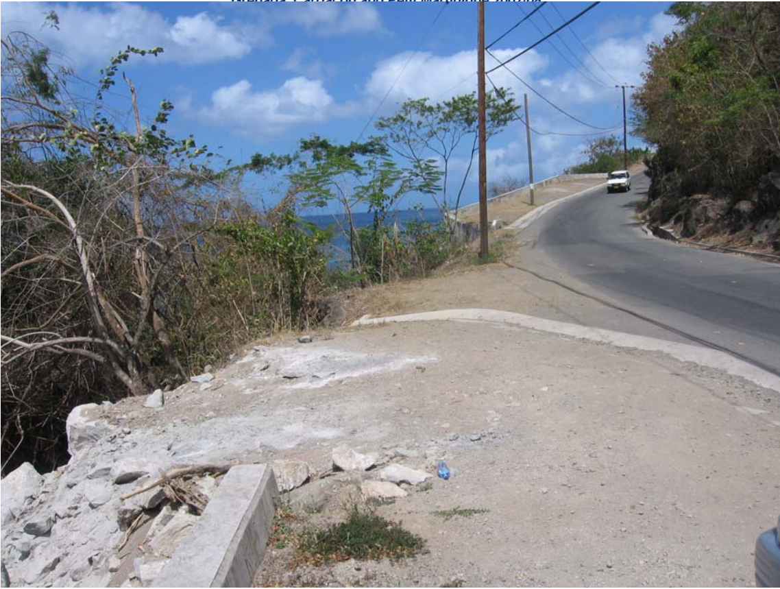
PHOTOGRAPH 11.1: SEA-WALL ALONG THE COAST
